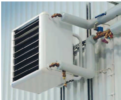
Fig.6.3.11 FHW fan heater with water coil
