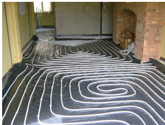
Fig.6.3.9 Radiant floor heating system
