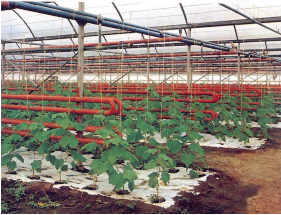
Fig.6.3.22 Aerial pipe heating system
